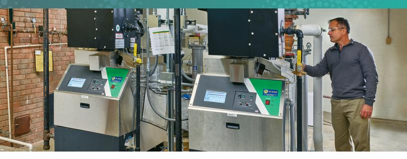
A boiler tune-up can improve boiler efficiency by more than 5%. It is recommended that a tune-up be performed annually by a qualified technician as part of a regular maintenance schedule. Besides saving energy and lowering operating costs, a boiler tune-up helps to:
