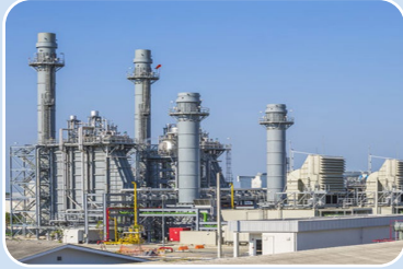
Combined Cycle Natural Gas
