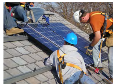
Crystalline solar modules mounted on aluminum racks, with airspace to keep them cooler.
