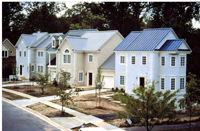
Flexible thin film solar panels blend in between the ridges of metal roofing.
