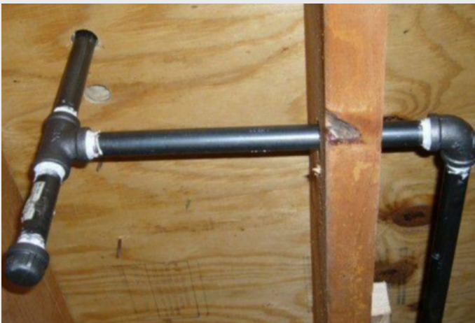
New black iron pipe, which is still used in some homes because of its durability.
