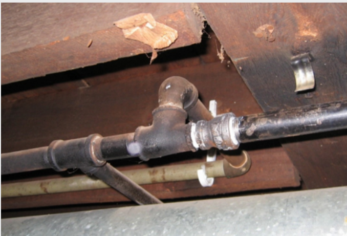
Old black iron pipe, which was used to deliver natural gas to homes from 1907 to the late 1970's.
