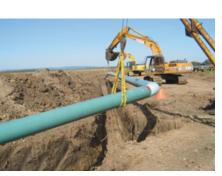
The pipe bending crew will use a bending machine to make slight bends in the pipe to account for changes in the pipeline route and to conform to the topography.
