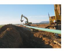
Lowering the welded pipe into the trench demands close coordination and skilled operators. Using a series of side-booms, which are tracked construction equipment with a boom on the side, operators simultaneously lift the pipe and carefully lower the welded sections into the trench. Non-metallic slings protect the pipe and coating as it is lifted and moved into position.
