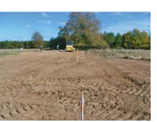
Once the pipe has been placed into the trench, the trench can be backfilled. This is accomplished with either a backhoe or padding machine depending on the soil makeup. As with previous construction crews, the backfilling crew takes care to protect the pipe and coating as the soil is returned to the trench. The soil is returned to the trench in reverse order, with the subsoil put back first, followed by the topsoil so that the topsoil is returned to its original position.
