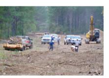
First, the survey crew carefully surveys and stakes the construction right-of way so that only the pre-approved construction workspace is cleared. Then, the clearing and grading crew leads the construction spread. This crew is responsible for removing trees, boulders and debris from the construction right-of-way and preparing a level working surface for the heavy construction equipment that follows.
