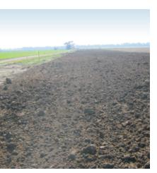
The final step in the construction process is restoring the land as closely as possible to its original condition. Depending on the project's requirements, this process typically involves decompacting the construction work areas, replacing topsoil, removing large rocks that may have been brought to the surface, completing any final repairs to irrigation systems or drain tiles, applying soil amendments, restoring fences, etc.
