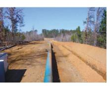
The trenching crew will use a wheel trencher or backhoe to dig the pipe trench in which the pipeline will be installed. The depth of the trench can vary across the entire pipeline to accommodate site-specific design criteria, pipe diameter and overburden requirements. The typical minimum depth for the pipeline will provide for 36 inches of cover above the top of the pipe, but the pipe will be buried even deeper at stream and road crossings.
