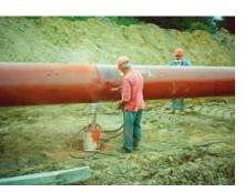
Line pipe is externally coated to inhibit corrosion by preventing moisture from coming into direct contact with the steel.
