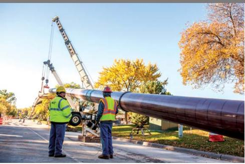
As part of the Metro Belt Line Project, CenterPoint Energy is replacing more than 60 miles of aging, large-diameter pipeline in the Twin Cities area.
