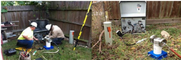
URD Cable Modernization
