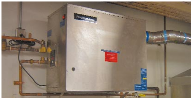
Using a natural gas booster water heater, such as this one by Precision Temp, instead of an electric booster, will save money and reduce your carbon footprint.
