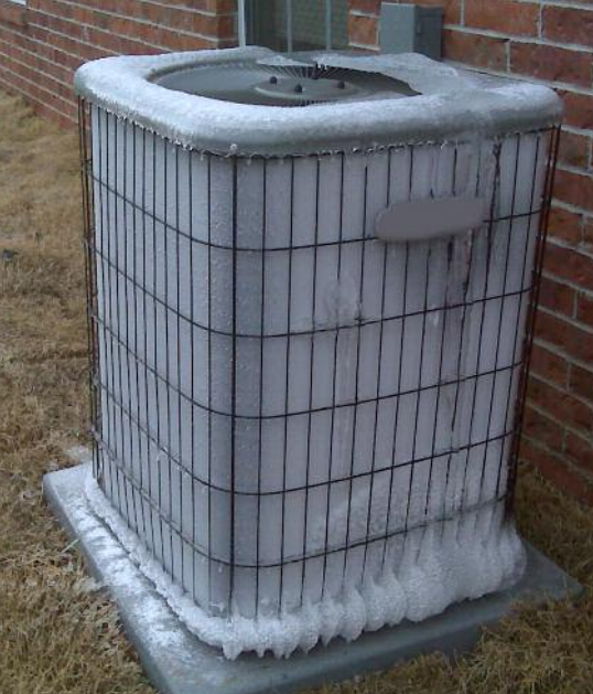
Air-source heat pumps are not effective below 32 F, as they require a substantial amount of defrosting cycle time – making them less efficient.
